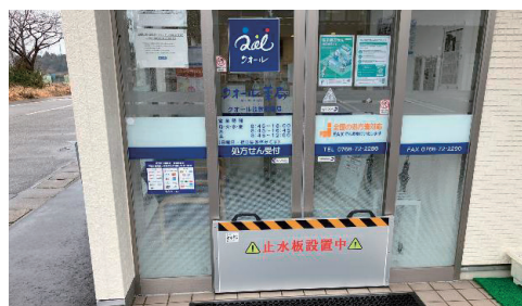
Water stop installed at the entrance to a pharmacy
